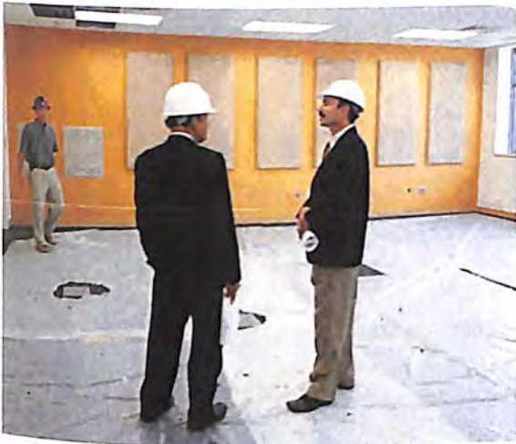
Dr. Varkey Titus, dean of the School of Business, center, and Dr. Alex Koohang, dean of the School of Information Technology, right, check out a second-floor classroom. The wall behind David Sims, director of Plant Operations, left, contains acoustical panels.
