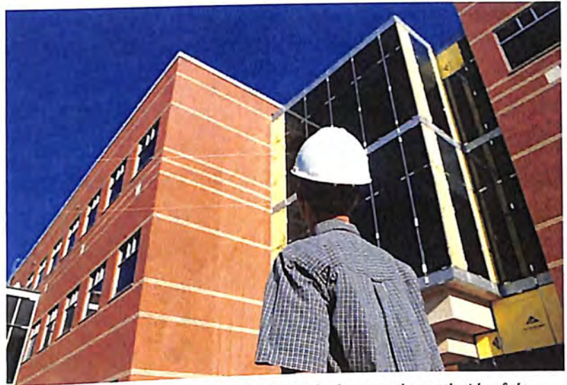
Sims stands in what will be a courtyard as he looks up at the south side of the Professional Sciences Building.
